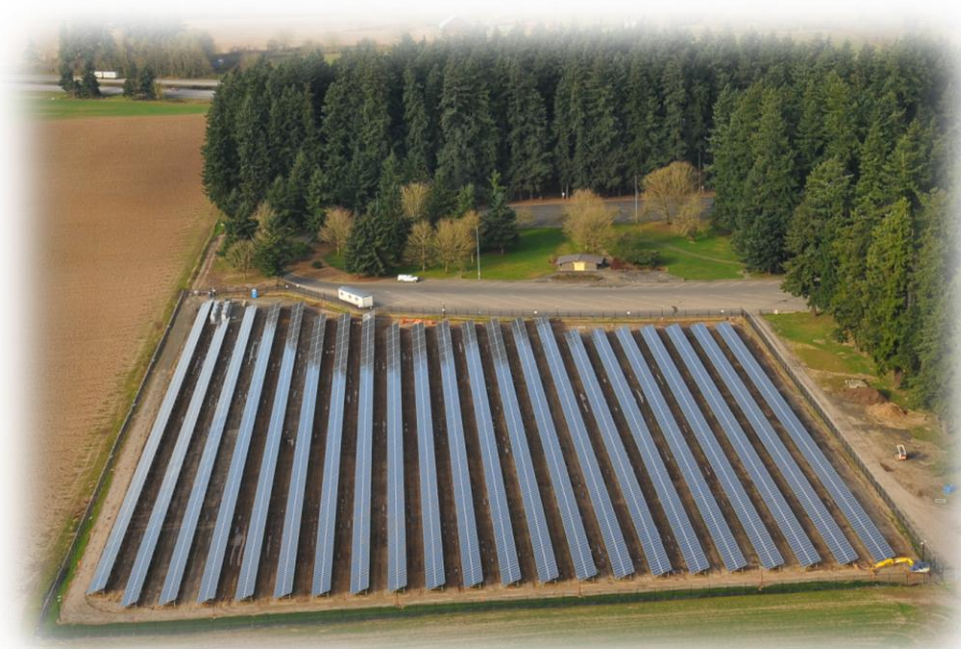
Baldock Solar Highway Project 1.75 MW Portland General Electric Oregon Department of Transportation
