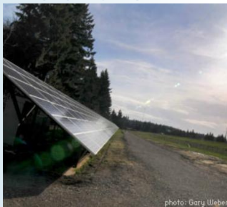
Sunway Solar Highway Project 104 kW
