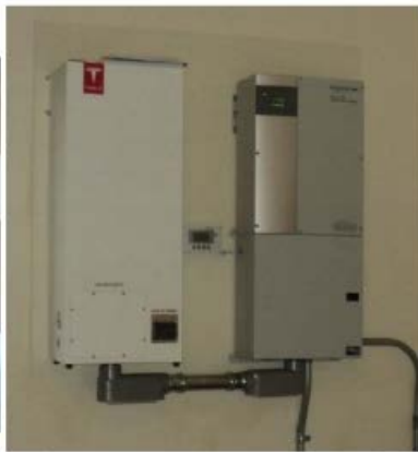
PV: 5.5 kW-CEC Storage: 5 kW / 10 kWh AC Li-ion
