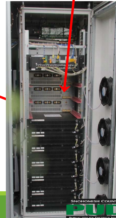
Inverter Power Stack
