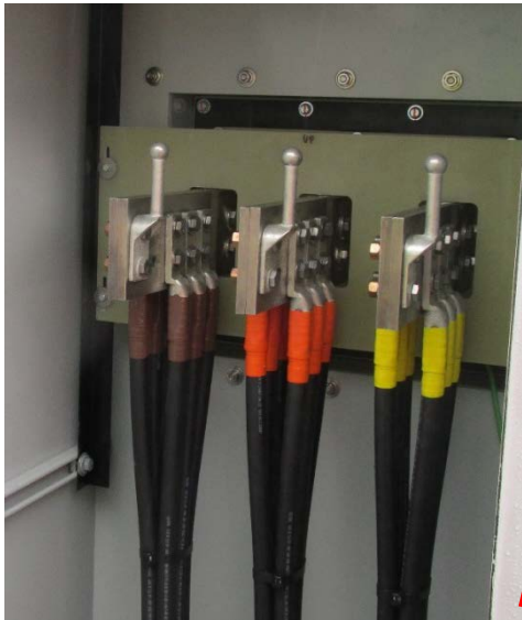
AC Connections And Breaker
