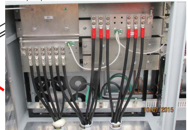
DC Battery Power Connections
