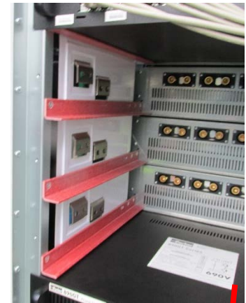
Inverter Power Stack
